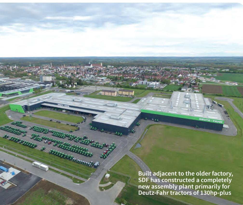
Built adjacent to the older factory, SDF has constructed a completely new assembly plant primarily for Deutz-Fahr tractors of 130hp-plus
